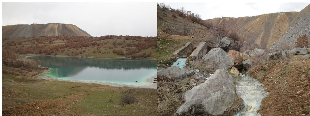
Fig. 2. Buchim Lake (left) and Buchim Dol (formation of Buchimski Dol, joining of collector and drainage waters under the mine waste dump, right)
