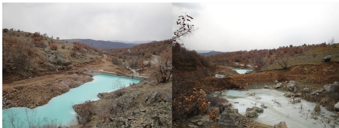
Fig. 3. Accumulation dam D1 (left) and earthen dam above the dam D1 (right)
